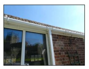
building. These rainwater fittings appear to have been renewed in recent years and show no signs of disrepair. The downpipes discharge rainwater below ground level.
