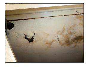
This hole in the roof has also caused significant damage to the asbestos fibreboard ceiling above and this needs to be replaced. Elsewhere these asbestos ceilings are in a reasonable condition commensurate with age, but replacement of ceilings containing asbestos fibres is an expensive and difficult
