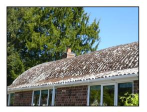
building is to be retained the roof coverings need to be completely stripped and renewed within the next few years.
