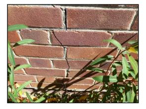
The building is exhibiting signs of previous movement, although appears currently stable. There is some cracking which has opened up within the external brickwork, notably towards the front of the lefthand elevation and I understand this has opened up within the last five years or so. There is also some outward
