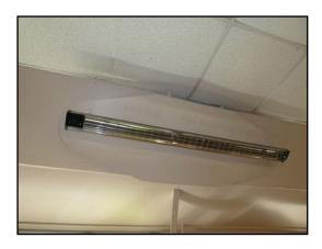
There is no heating within the kitchen or the toilet and the only heating within the main hall is from ceiling mounted electric heaters. These will prove highly inefficient as heat rises and the vast majority of the heat generated will disappear through the roof above. See related comments below.
