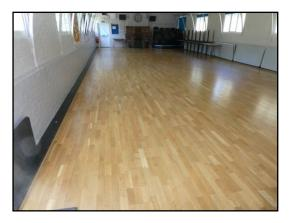
The floor is of a solid construction, probably built in concrete and with a cement screed although the floor is concealed by internal floor coverings.
