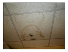
The suspended ceiling is in a reasonable condition although will require ongoing maintenance, including where rainwater ingress has caused dampness and individual tiles need to be replaced. This is currently evident to one tile in the kitchen which is damp and damaged due to rainwater ingress above through a hole in the roof.
